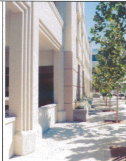
Architectural detailing on a parking structure.
