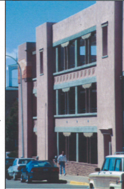
Accent material used to add color and relief to a parking structure wall.
