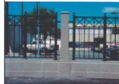
Concrete block in combination with metal fencing.
