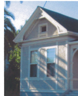
Italianate window with framing and surrounds
