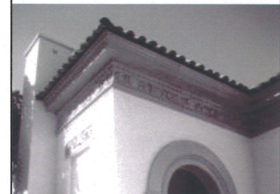
Roofs should include cornices or other detailing appropriate to the architectural style of the building.
