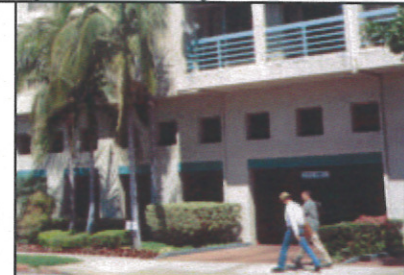
Garage entrances should be recessed from the front façade of the building.
