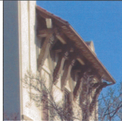
Brackets and supports beneath a Downtown roof.
