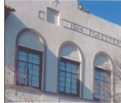
Windows should be inset from wall surface.
