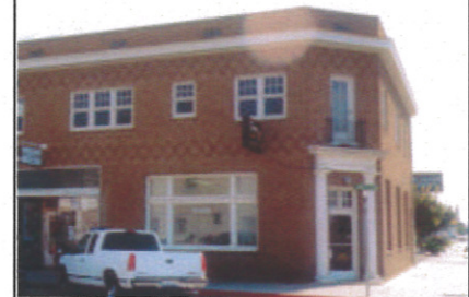
Location of a corner entrance.
