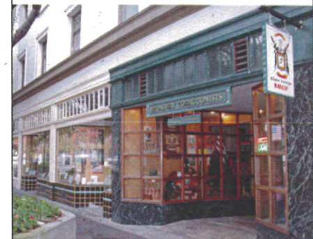
Clerestory windows above storefronts.
