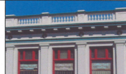
Straight parapet with railing detail and cornice.
