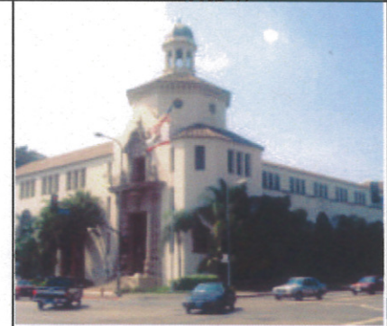
Prominent treatment at a highly public intersection.
