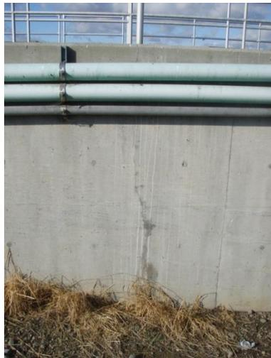
*Potentially Leaking Crack at Chlorine Contact Tank*
