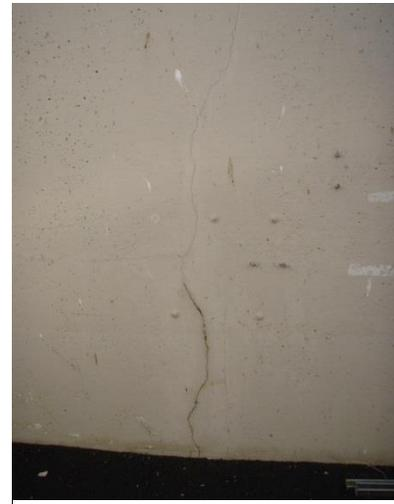
*Potentially Leaking Crack at Tertiary Filters/Flocculation Tank*
