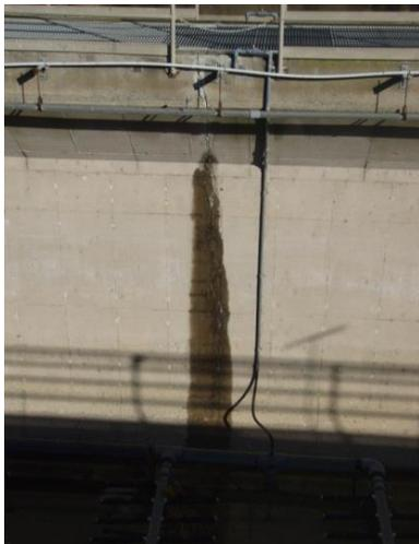
*Leaking Crack at Aeration Basin*
