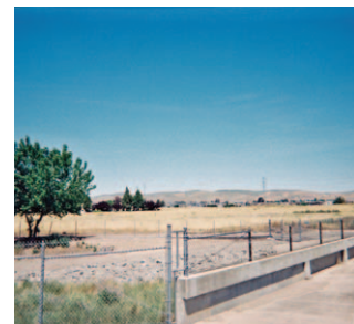
Arroyo Seco Flood Channel.
