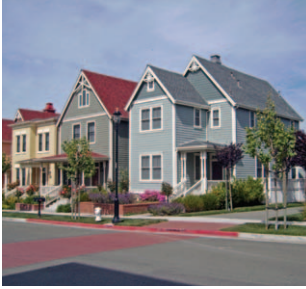
These roof forms and pitches are consistent with the traditional style of the homes.
