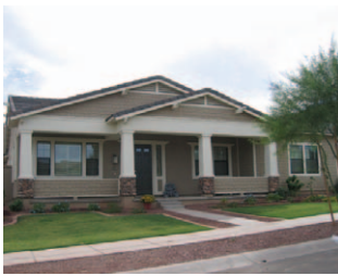
Porches are used as the transitional element to create interest and variety in the front elevation
