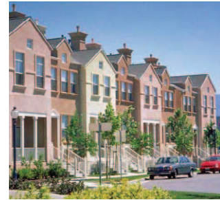
Multi-unit buildings should be designed with distinctive individual units within, with each including a legible street facing entry.
