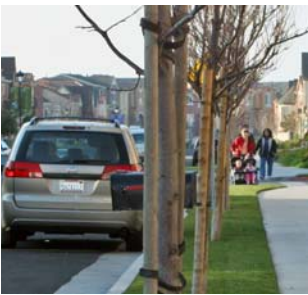
Parallel on-street parking spaces are provided on the Arroyo Vista Site.
