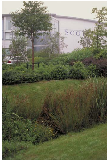
A natural swale will run along the both sides of Jack London Boulevard, serving as a functional element for the stormwater management system as well as a design element meant to enhance the entry corridor.
