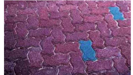
Pavement made from recycled tire rubber.
