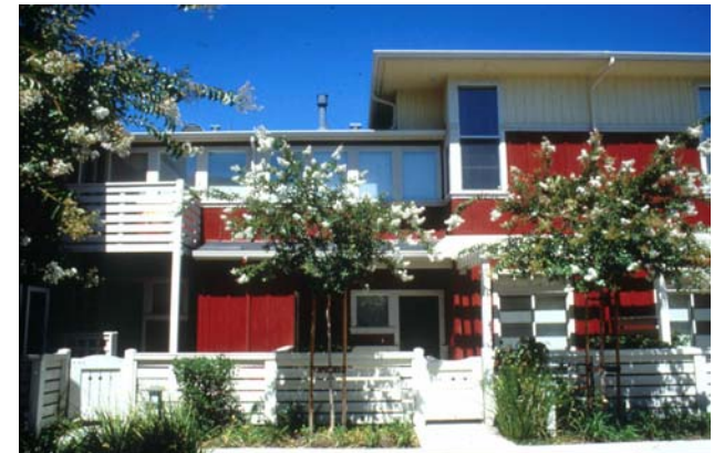
Street-facing façade is detailed with trellis, roof overhang, window trim and an overall color palette that enhances architecture.
