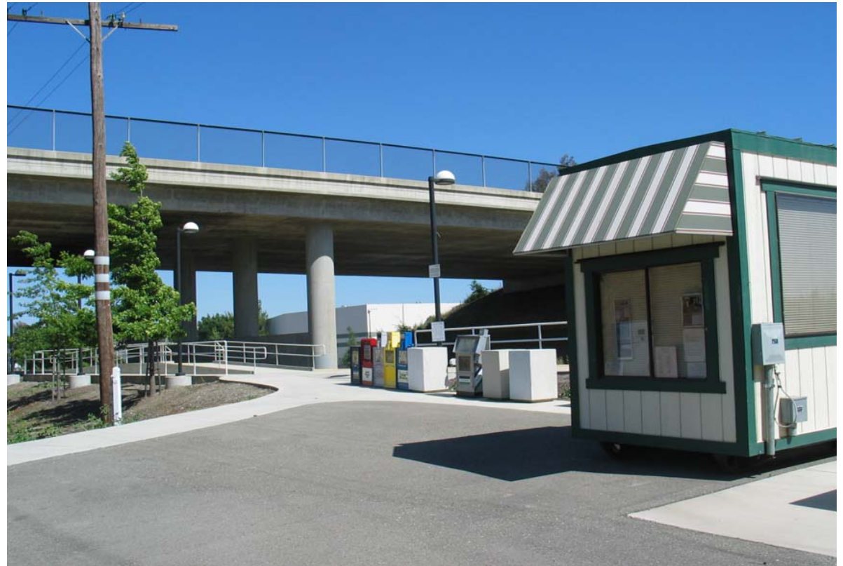
View from the commuter parking lot on the west side of Vasco Road toward the underpass leading to the ACE platform.
