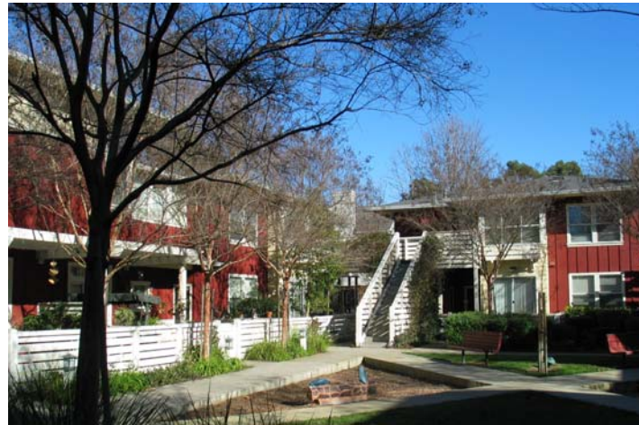
Community open space functioning as an extension of private open space areas for all units.
