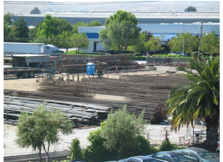
The Brisa site is surrounded predominantly by light industrial uses.
