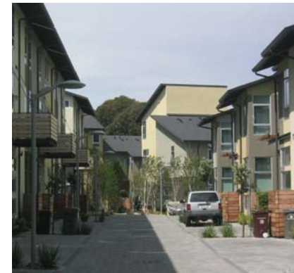
Alley landscaping helps soften the spaces between buildings.
