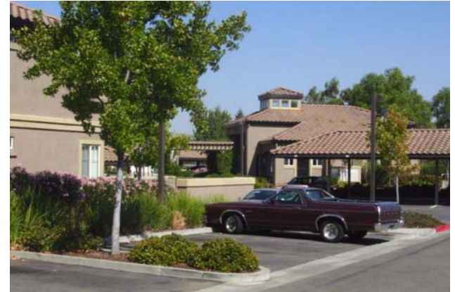
Landscaped parking area for multi-family residential development.
