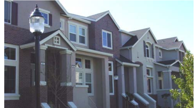
Roof designed as part of the building.
