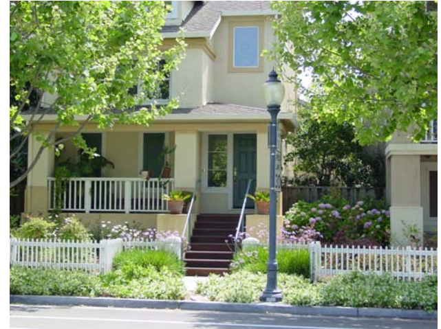
Entry areas facing public streets shall be adequately landscaped to soften hard edges and screen views.
