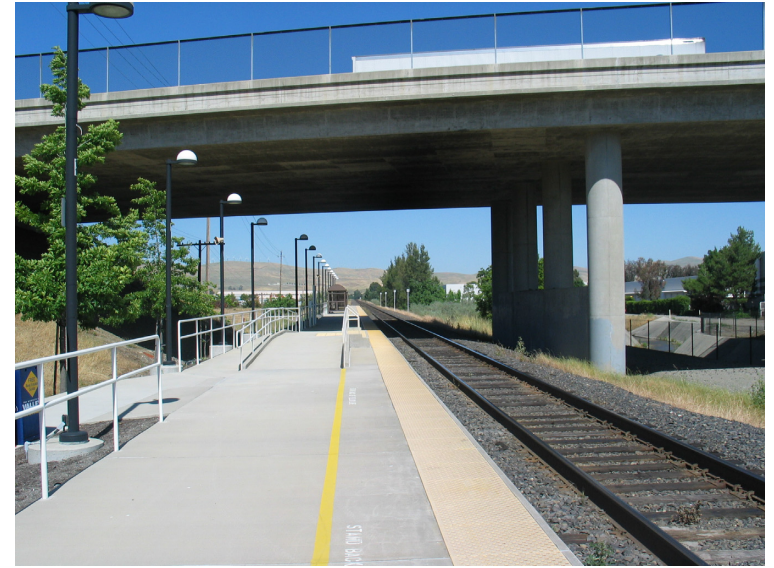
The ACE platform and Vasco Road overpass, viewed eastward from the west side of Vasco Road.
