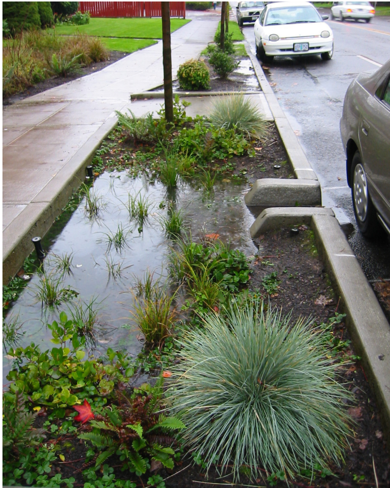
Well-integrated water run-off systems.
