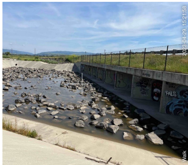
Figure 3: Large Drop Structure and Culverts Downstream of Airport
