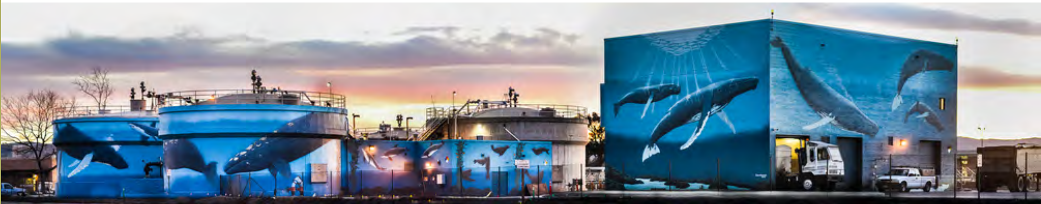
Whale murals by artist Darren Greenwood, located at the Livermore Water reclamation plant in 2010.
