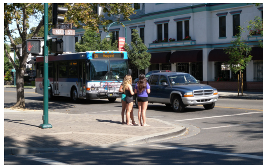
Bulb-outs shorten the walking distance across intersections, improving pedestrian safety.
