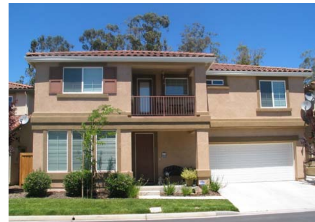
Garage is set back from front façade to emphasize front entry to residence.
