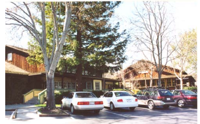
Landscaped planter strip with disabled access ramp is the width of a parking space.
