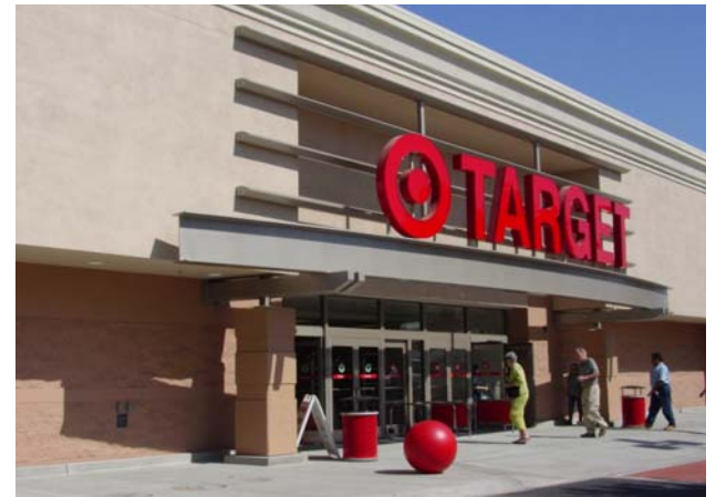
Individual three dimensional letter sign mounted on awning structure.
