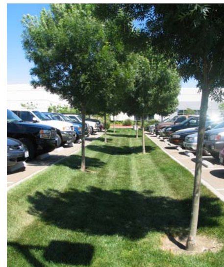
Drainage swales for parking lot runoff reduce negative impact on overall water quality.
