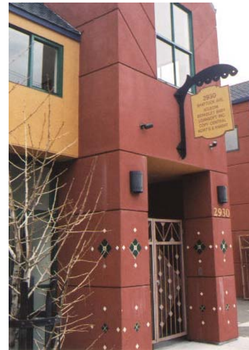
Upper floor entrance marked by greater building mass.
