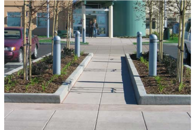
Bollard lighting for pedestrian path.
