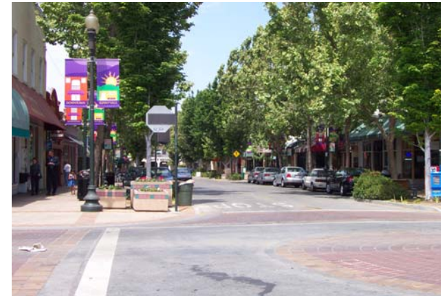
Pedestrian traffic lane crossing with textured paving material.
